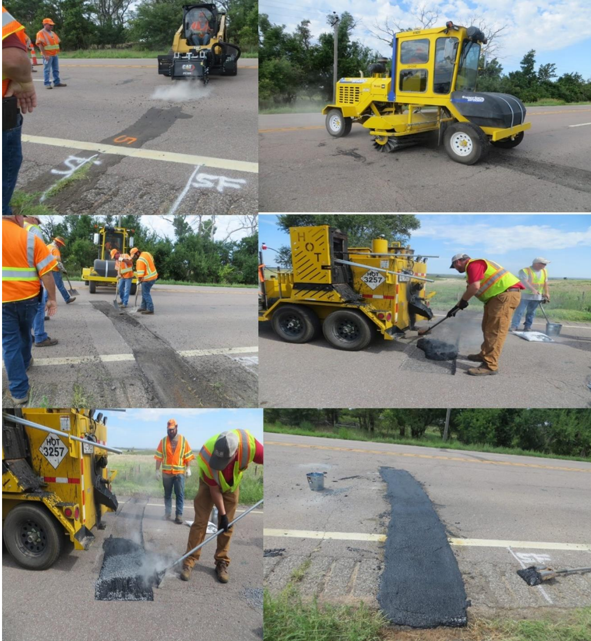
Figure A.1 Repair Activities of Crack #5
