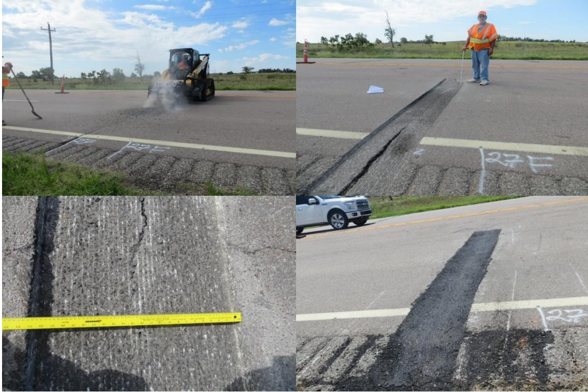
Figure A.6 Repair Activities of Crack #27
