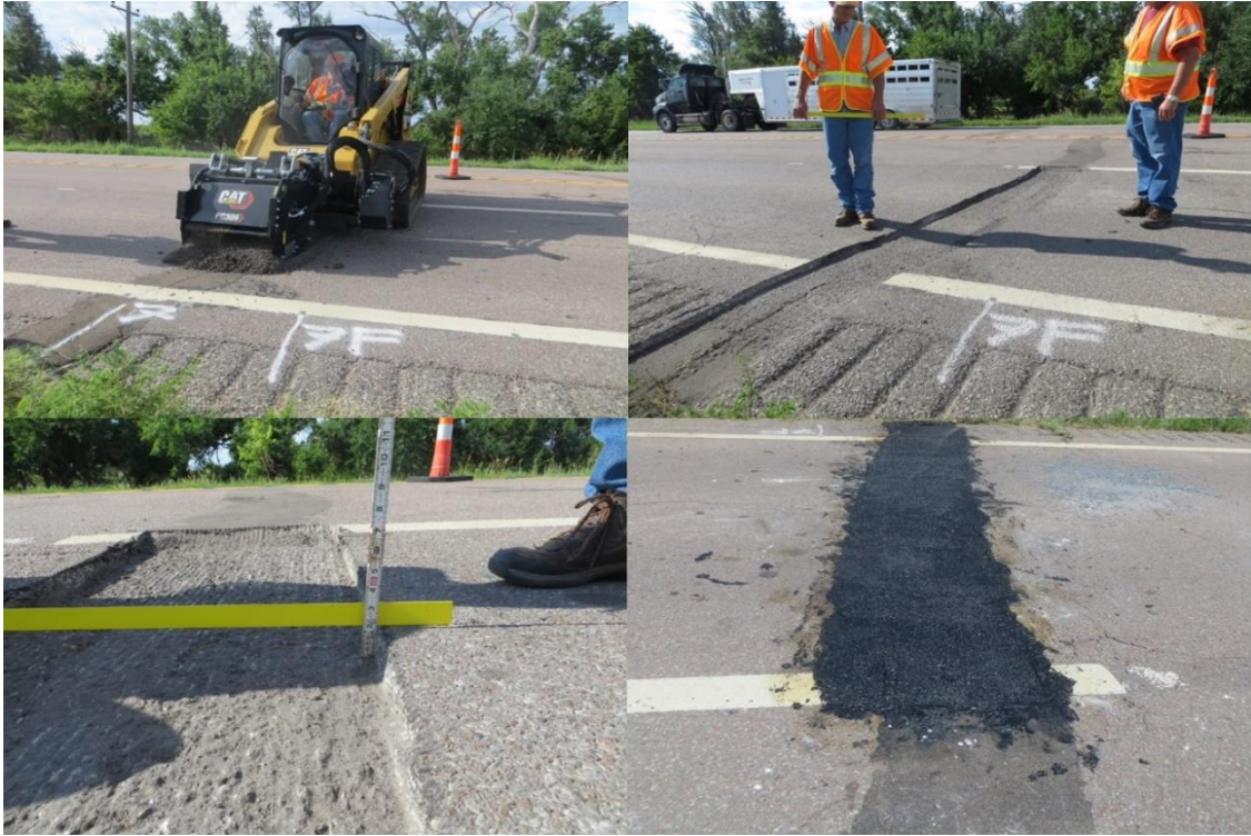
Figure A.2 Repair Activities of Crack #7
