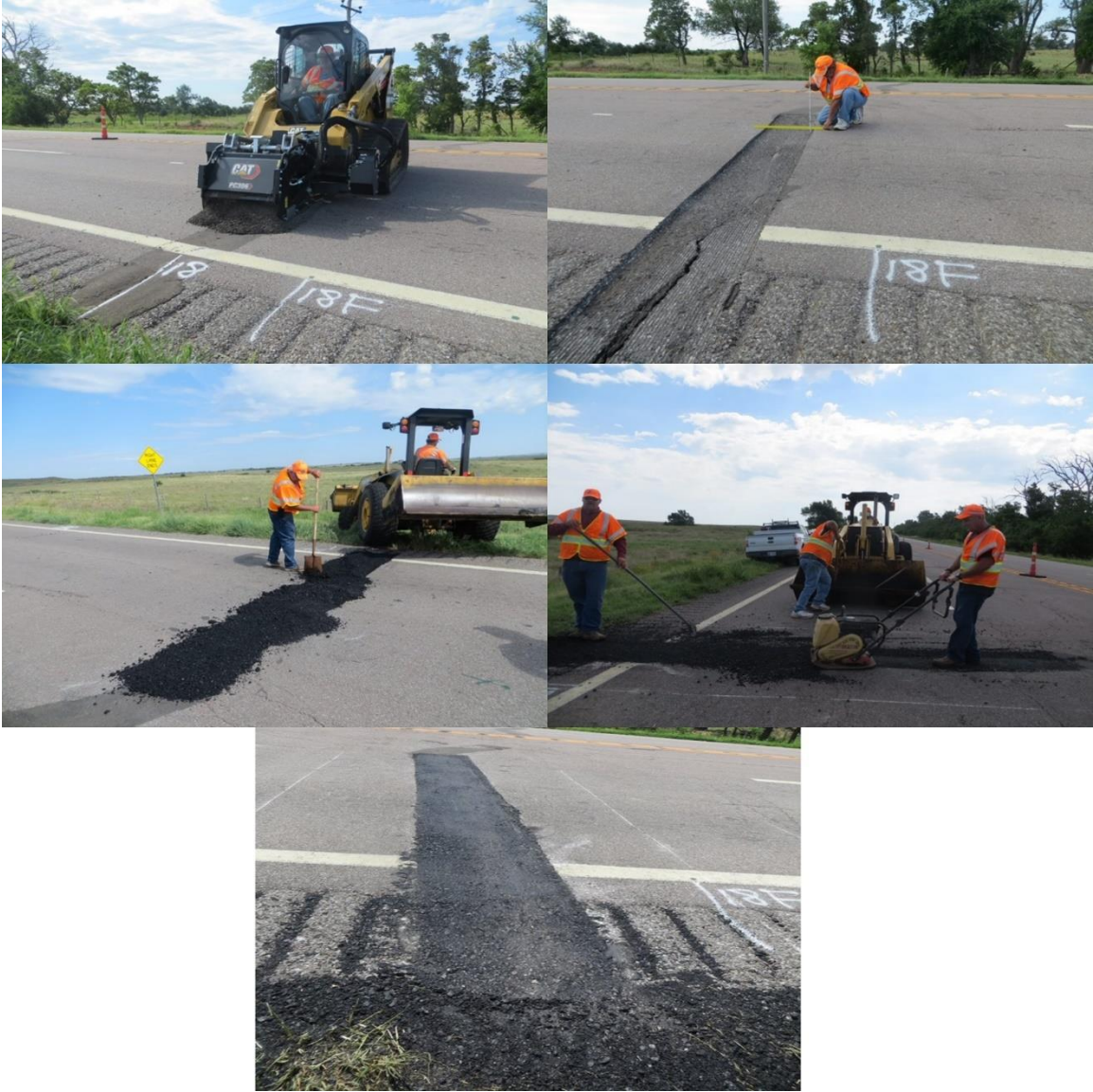
Figure A.5 Repair Activities of Section #18
