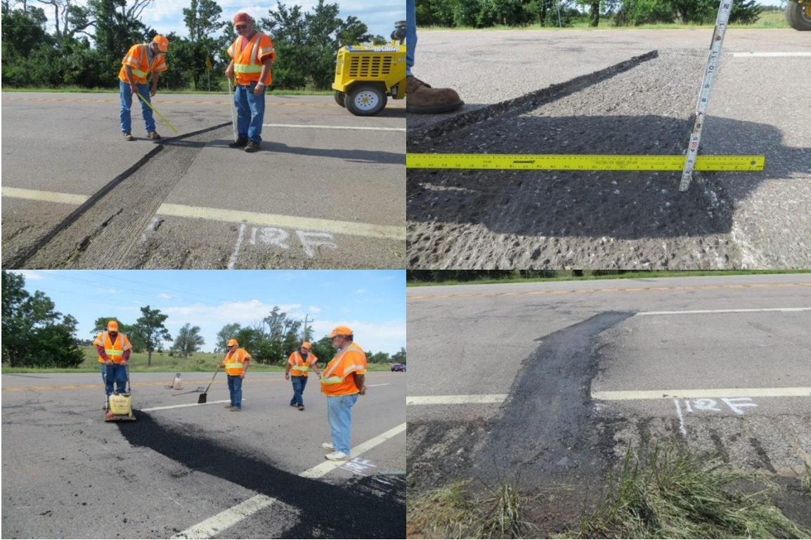
Figure A.4 Repair Activities of Crack #12
