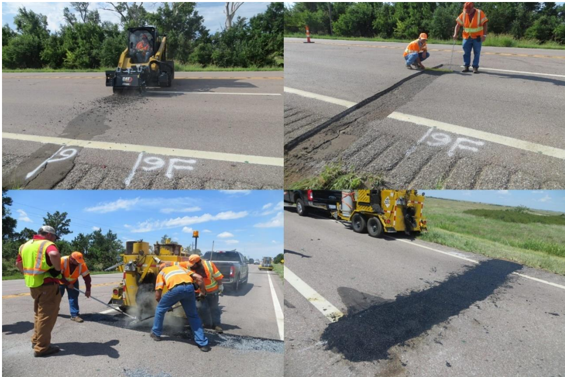
Figure A.3 Repair Activities of Crack #9
