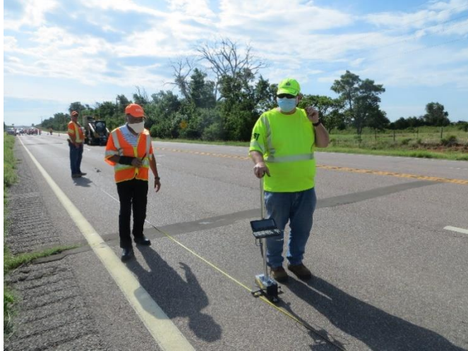
Figure 2.7 Face Dipstick measurement in US-270 test site
