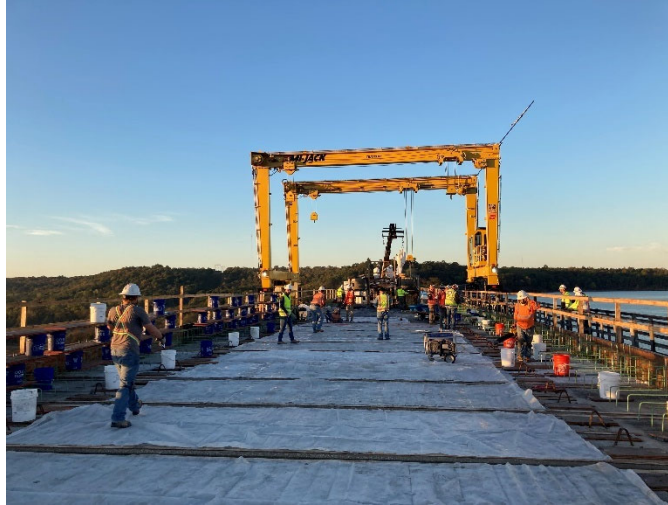
Figure 35. Spans 8 and 9 ready for UHPC joint placement
