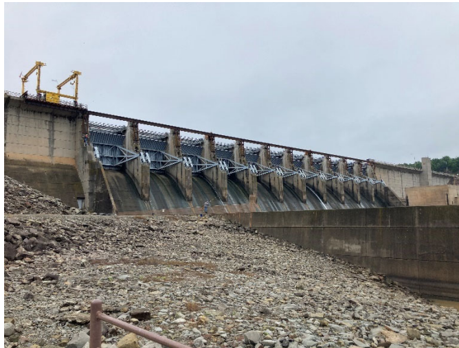
Figure 1. Lake Eufaula spillway after demolition of existing bridge
