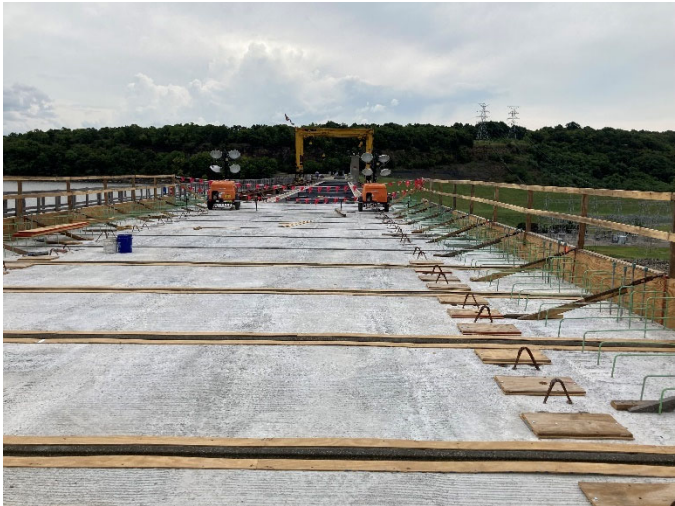
Figure 25. Bridge deck immediately before Span 1 joint placement
