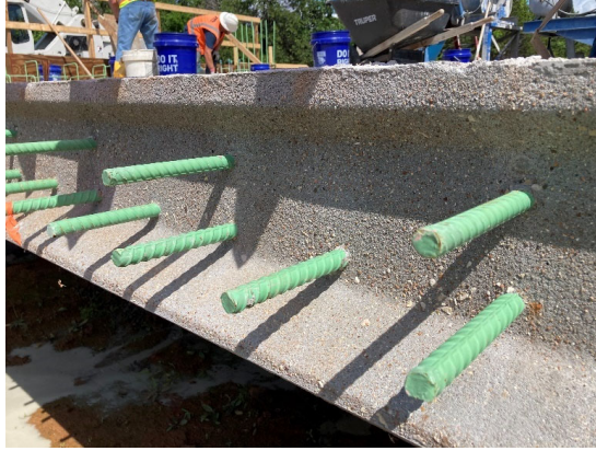
Figure 3. Close up of joint exposed aggregate surface and epoxy coated bars
