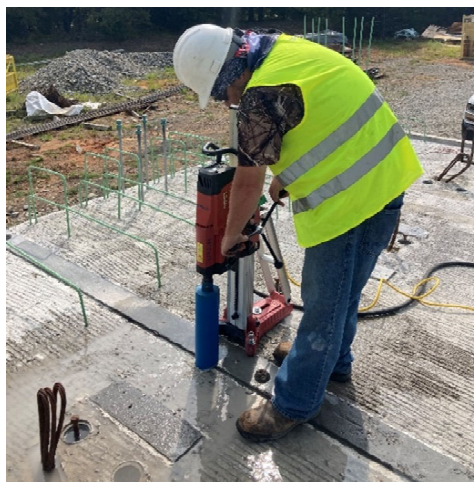
Figure 19. Coring of the bridge mock-up at the joint interface
