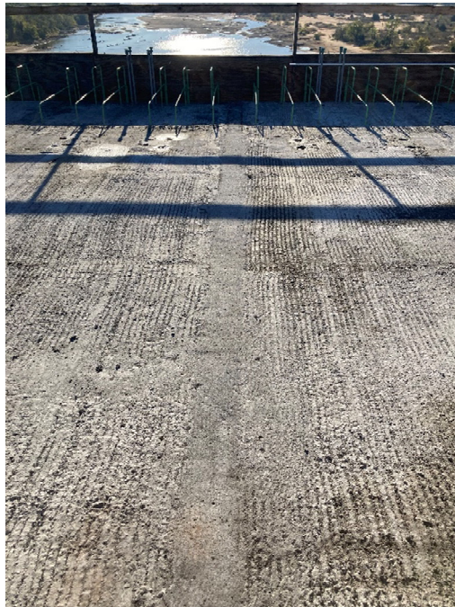
Figure 38. Example completed UHPC joint
