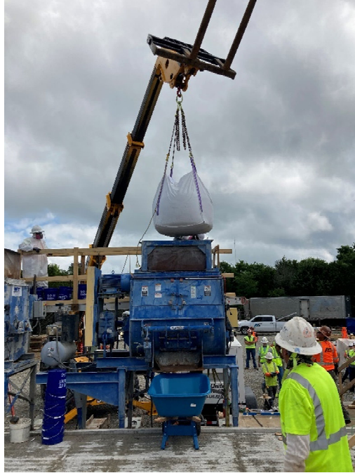
Figure 8. Placement of the UHPC premix into one of the stationary mixers
