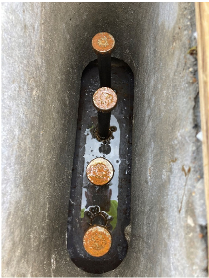
Figure 4. Shear studs visible in one of the mock-up shear pockets
