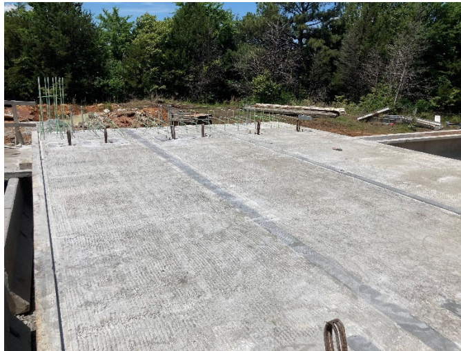
Figure 2. Overall view of the bridge deck mock-up
