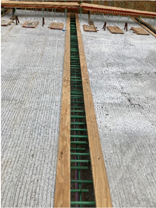
Figure 26. Joint prepared for casting and showing splice reinforcement
