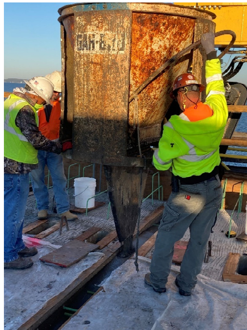
Figure 36. Placement of UHPC using the concrete transfer bucket and rubber sleeve
