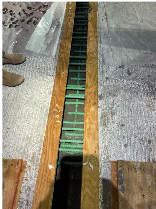
Figure 33. UHPC in one of the joints on Span 1
