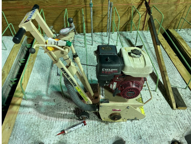
Figure 39. Grinder used for grinding UHPC joints
