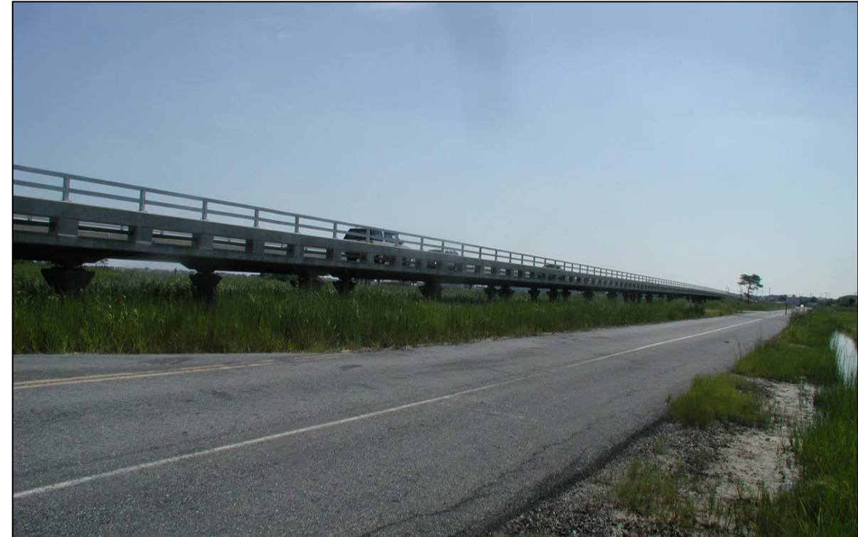
Elevation View of SR54 Viaduct From Old SR54 Alignment, Fenwick DE Cost = $16 M in 2001
