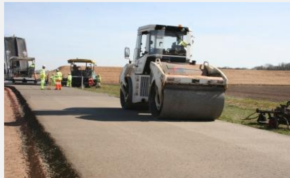
Roller Compacted Concrete (RCC)
