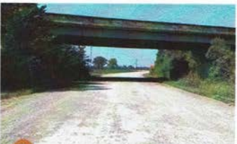
2 Reclamation in process
