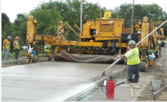
Conventional Concrete Pavement
