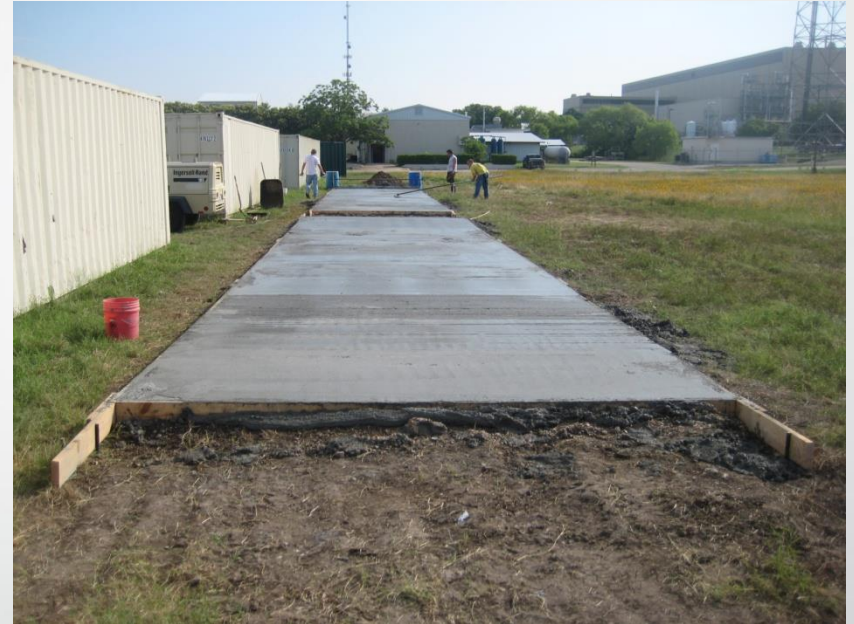
Slabs Prior to Hydro-demolition
