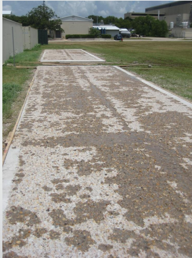
Completed Hydro-demolition
