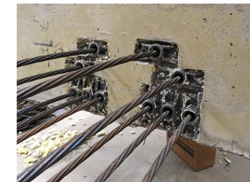
Formwork for the Web Section (Above) & South End Post-Tensioning Anchorage (Below)
