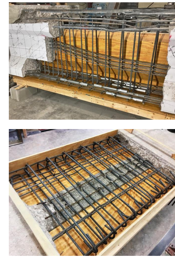
North End Girder & Deck Repair Reinforcing
