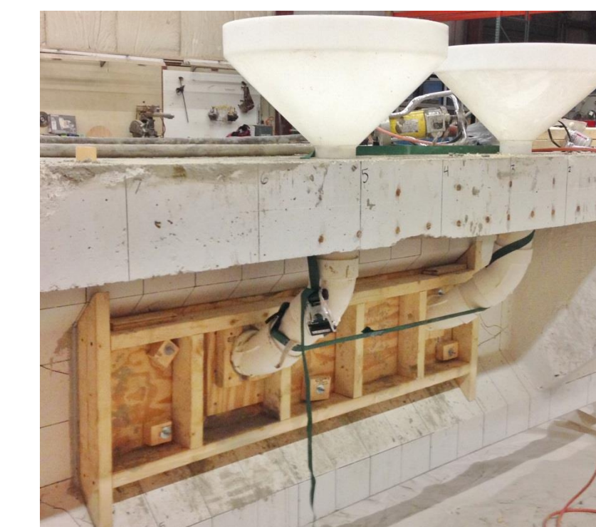
Formwork for the Web Section (Above) & South End Post-Tensioning Anchorage (Below)
