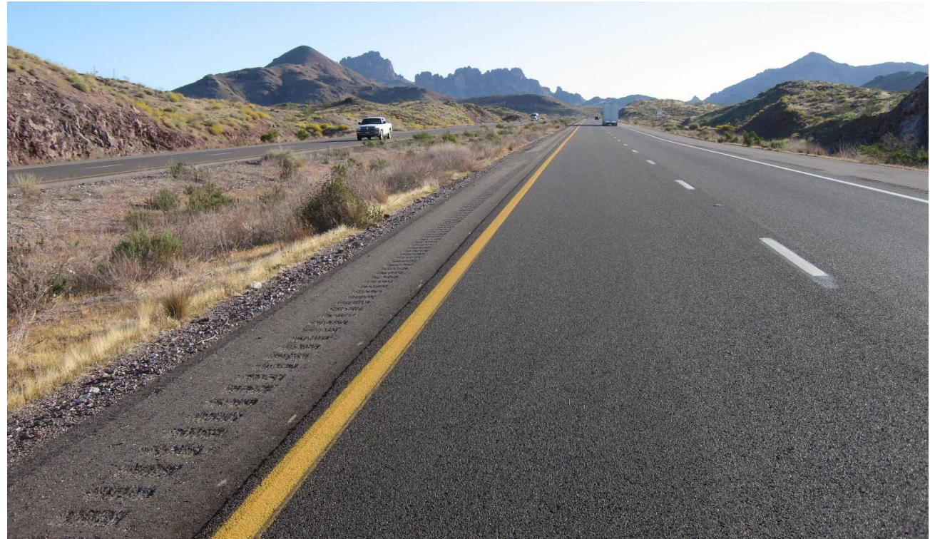
AR-ACFC on SR 64 east of Bullhead City, AZ.
