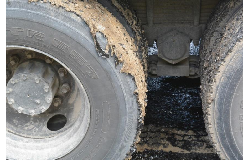
Tack pickup due to unclean roadway surface
