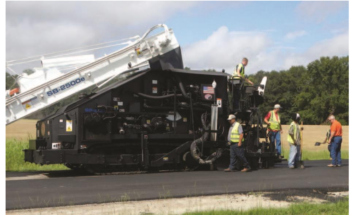
Spray paver being used on NCAT's Lee Road Pavement Preservation experiment.
