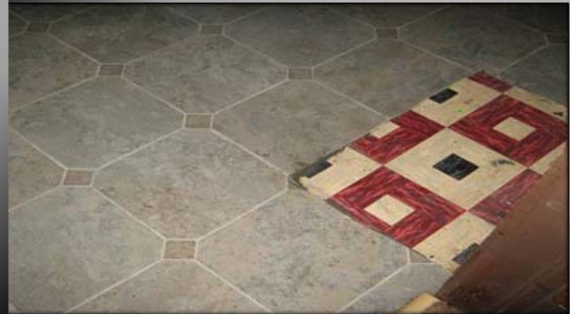
Old vinyl flooring >> Tiles Mastic
