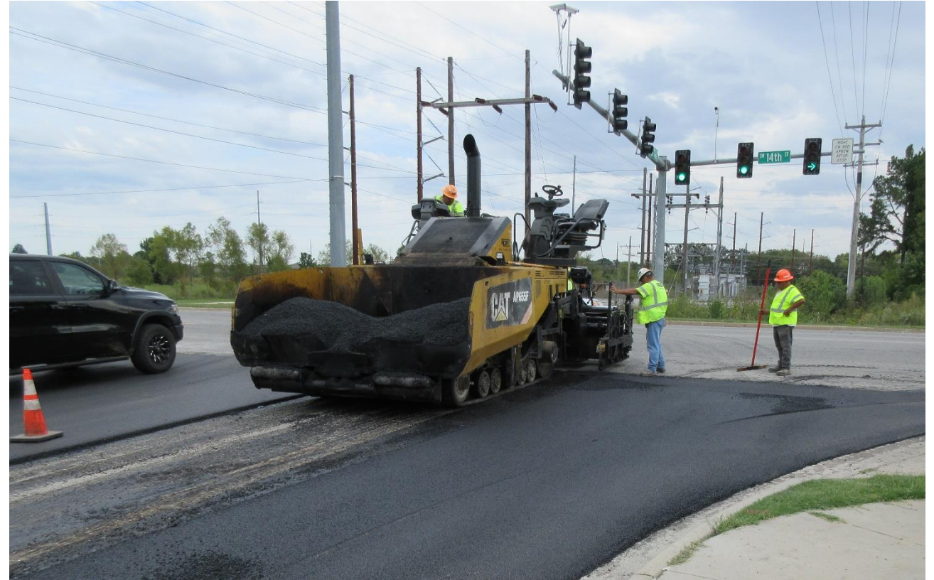
Asphalt being placed in NWA
