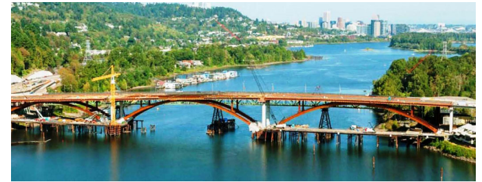
Sellwood Bridge – Multnomah County, OR
