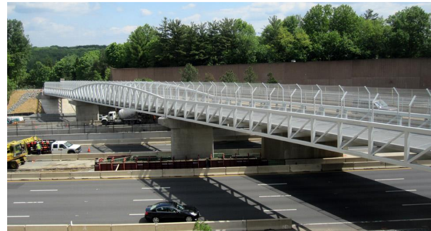
FRP Pedestrian Bridge in Virginia
