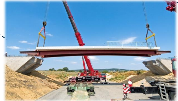
Bridge construction 2000s
