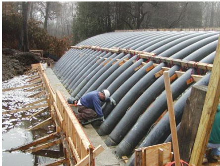
(composite arch bridge)
