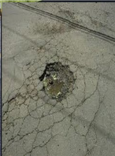
Cracks due to stripping
