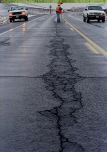
Cracks due to stripping
