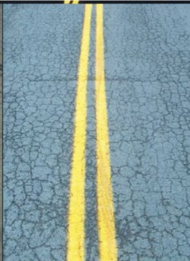
Fatigue cracking
